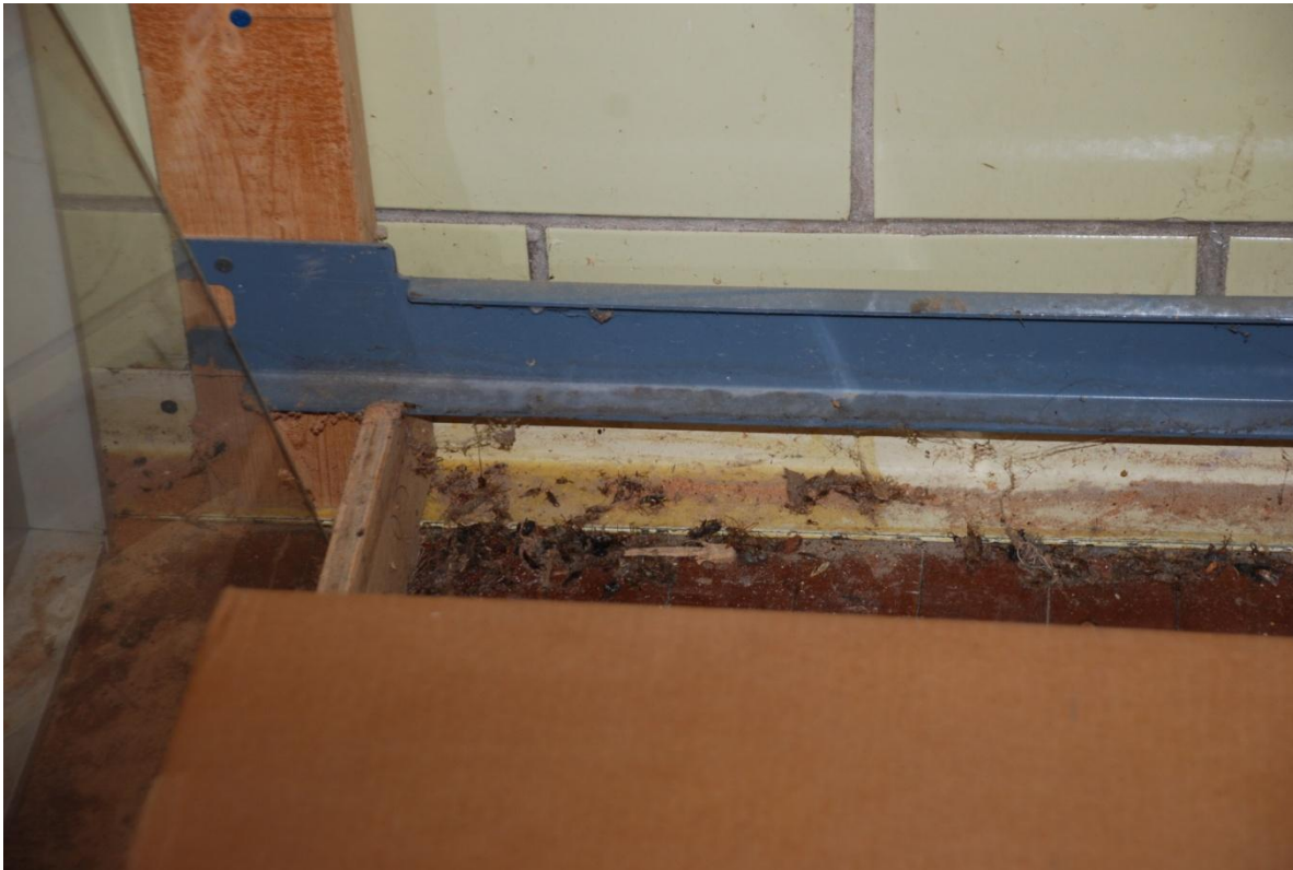
Figure 45: The space below the shelving in the northeast corner is a perfect pest haven..
