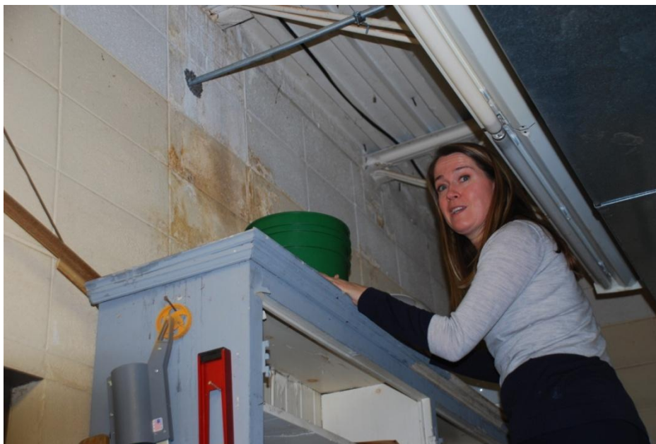
Figure 9: One of many buckets found in the Lincoln Center. Note the staining on the wall.
