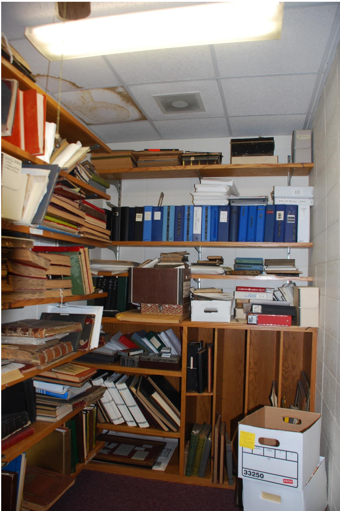
Figure 59: Archives room. Note staining on ceiling from previous roof leak.
