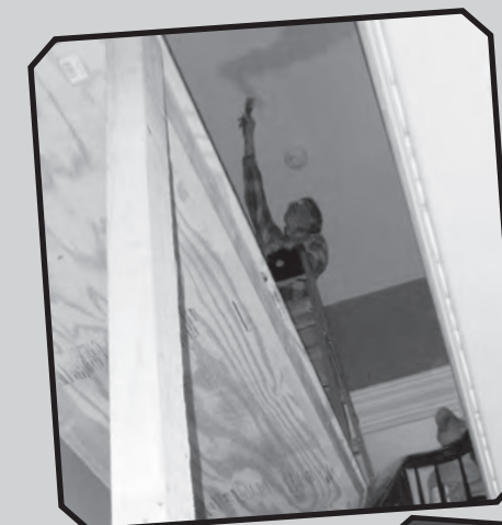
Greg Kaiser scrapes and patches peeling paint high above the beautiful staircase.
