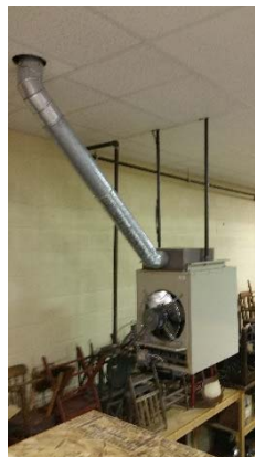
M-14 Unit Heater East and West
