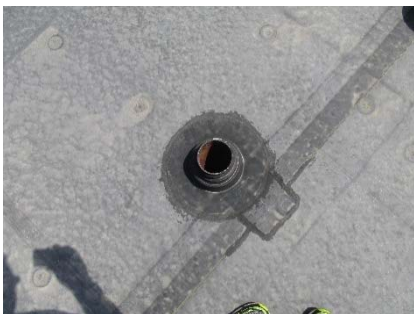
P-5: Cast iron roof vent pipe
