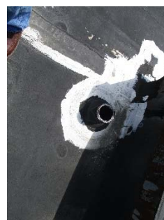
P-6: Cast iron vent pipe
