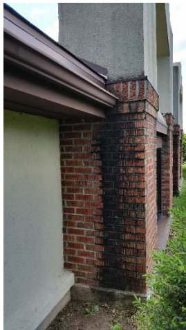
A-5: Improper flashing
