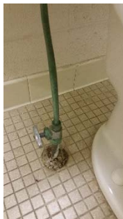
P-9: Deteriorating shut off valve
