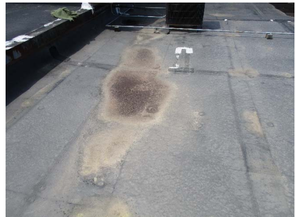
A-24: Water debris spotting
