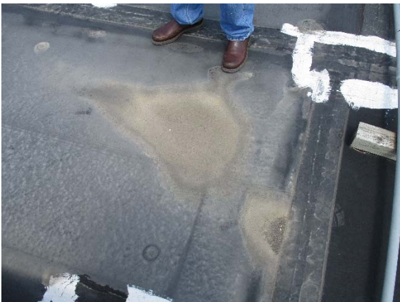
A-23: Water debris spotting
