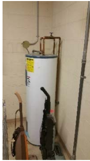
P-7: Electric water heater
