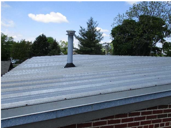
A-17: Screw down metal roofing
