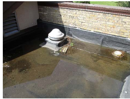
P-4: Roof Drain with built up debris
