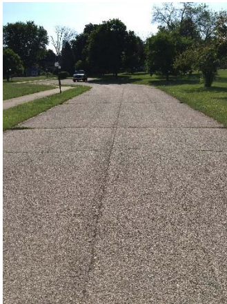
Figure 3 - Driveway Pavement Cracking
