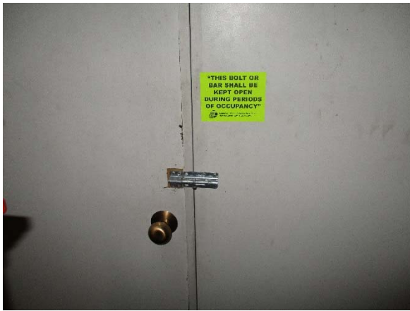
A-43: Non-compliant door hardware
