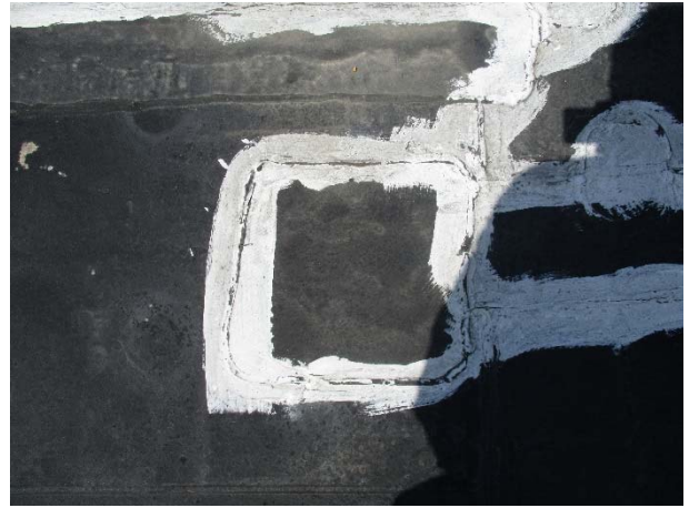
A-20: Roofing Sealant
