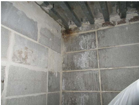
A-27: Water infiltration
