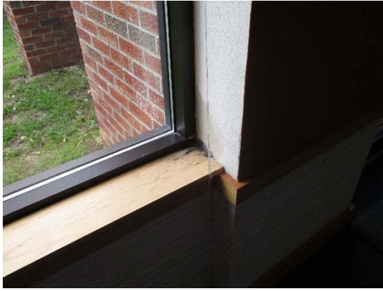
A-7: Water Infiltration
