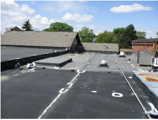
A-19: Re-roof (lighter is newer)
