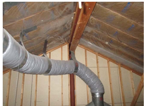
A-30: Attic Space with flex duct
