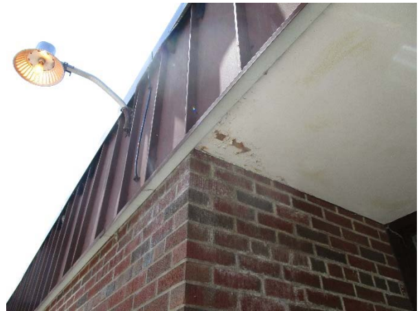
A-26: Efflorescence
