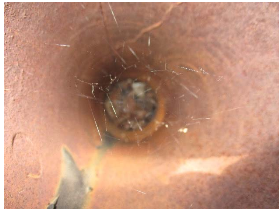
P-2: Roof vent with built up debris r
