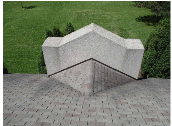
A-6: Roof drainage/ improper flashing
