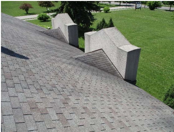
A-15: Shingle Roofing 1989 addition
