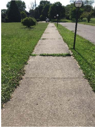
Figure 1 - Concrete Sidewalk Settling
