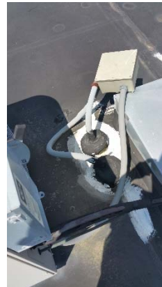
E-32 Roof Condenser Wiring
