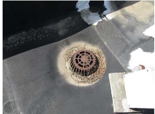
A-22: Debris at roof drains
