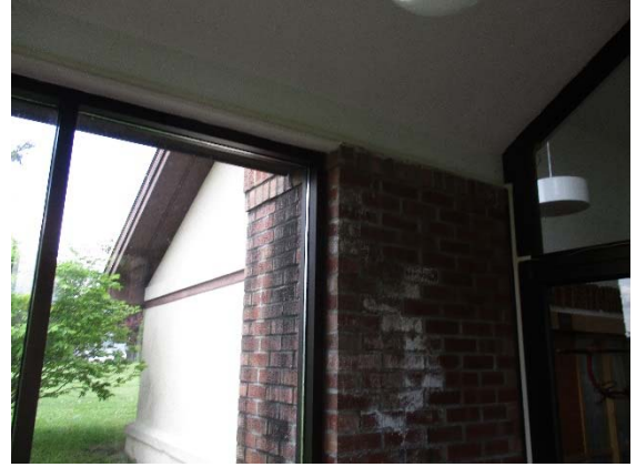
A-4: Water Infiltration
